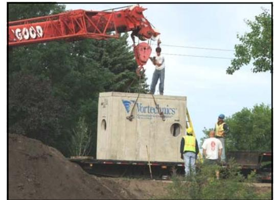
Installation of oil and grit separator to reduce nonpoint source discharge into the Au Sable River.
