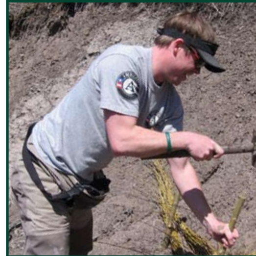
Nathan Skibbe (Huron Pines) pounds willow stakes to help restore the eroded slope at Claybanks on the Au Sable River.
